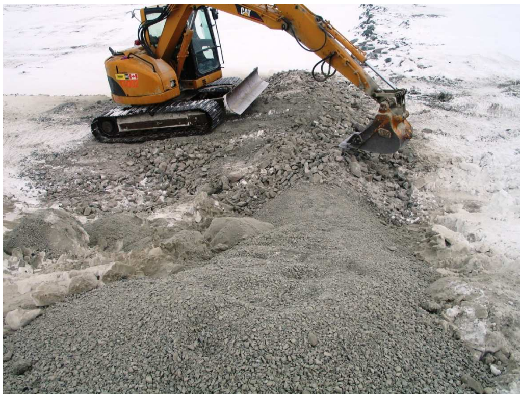
Photo 5: Cable covered with \frac{3}{4} in crush. Final ROQ surfacing underway.
