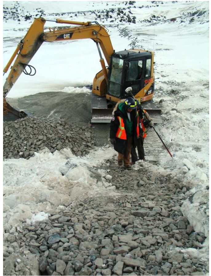
Photo 1: Surface of Pollution Pond bank after snow removal. Cable path between Pollution Pond floor and road. Photo 2: 6 in material placed to fill voids in rip rap .
