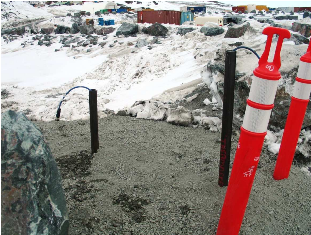
Photo 8: Finished product. The second pipe could have been higher. A wood junction box will be fastened to the pipe to protect the end of the cable.
