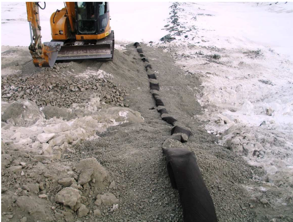
Photo 4: Wrapped cable ready for \frac{3}{4} in crush.
