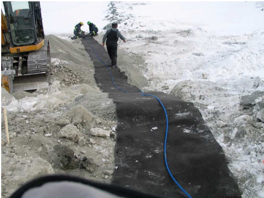
Photo 3: Preparing to wrap cable with geotextile.
